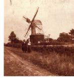
It was a post mill windmill, meaning it is an earliest type of European windmill. The feature is that the whole body of the mill that houses the machinery is mounted on a single vertical post, around which it can be turned to bring the sails into the wind.
